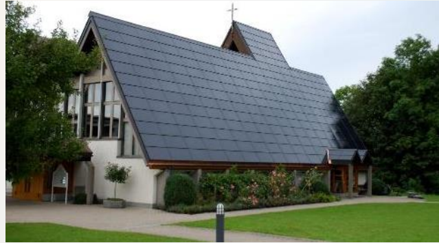
A roof that generates energy (solar panels replacing roof tiles)
