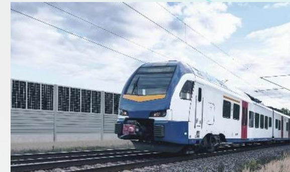
Noise barriers with integrated solar panels
